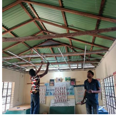
The new frame
