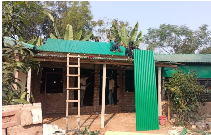
The extra class under construction
